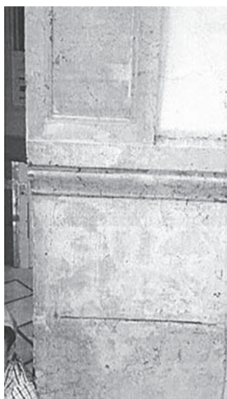
Figure 1. Color changes in the restoration material used in natural stone cracks on a facade (photo by Olga Smirnova in Malaga city center in 2019)
