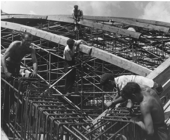
Figure 7. Construction of Hall 2 of the Belgrade Fair – assembly of the rebar for the edge arches and the structure of the shell (Source: https://sajam.rs/en/sanu-exhibition-dedicated-to-the-belgrade-fair-phenomenon-on-local-and-global-scale/# )
